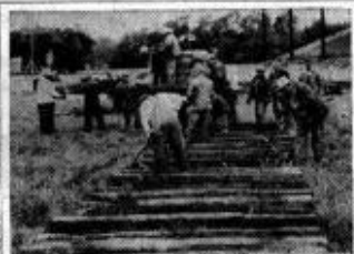
Laying Track at the Fairgrounds for 'Cyrus Halliday'
